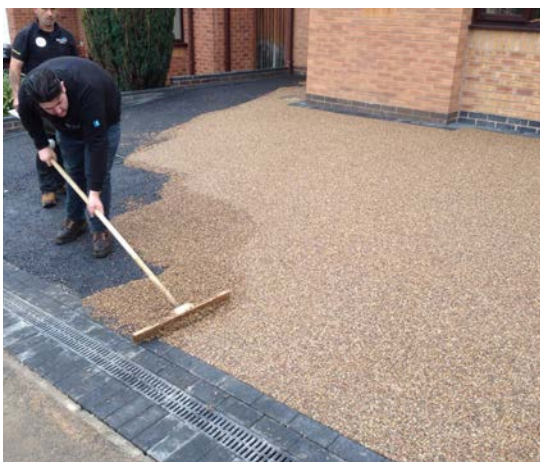
ABOVE: Resin bound paving construction and granite edging sets
